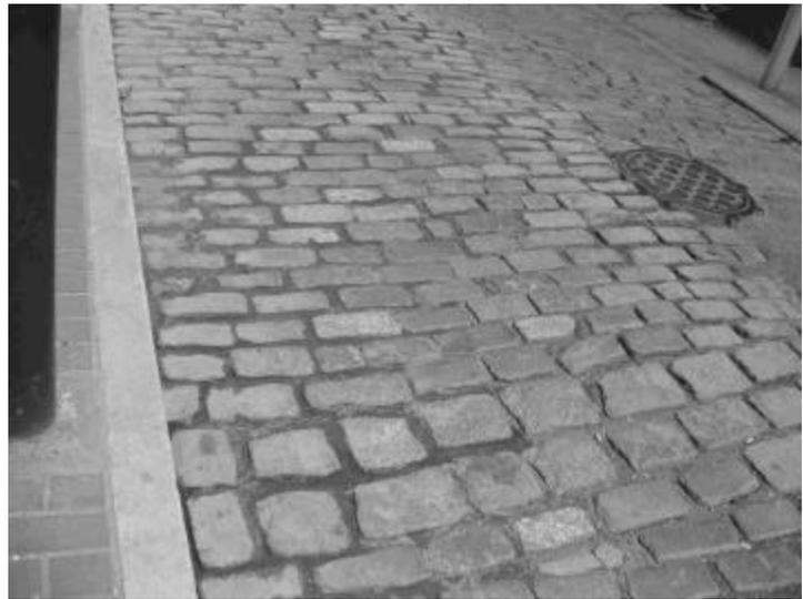
**Figure 9: Paving types; notice the two rows of Belgian Blocks in the foreground**
